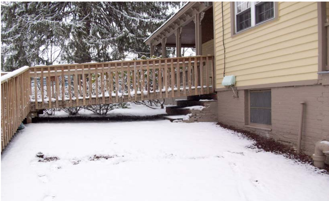
6) View of the vent pipe and fill port associated with the 1,000-gallon fuel Oil Tank.
