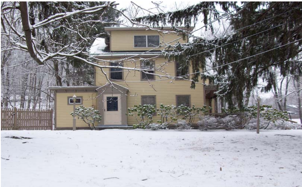
2) Another view of the front of the commercial/residential building on the Property.
